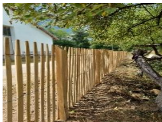
Cleft paling H 1,5 m Square stake 7 × 7 cm
