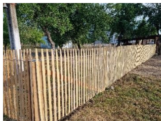
Cleft paling H 1,5 m Spacing 3–4 cm
