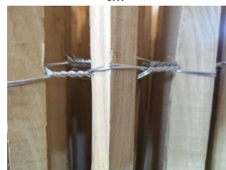
Cleft paling Galvanised wires \varnothing 1,8 mm
